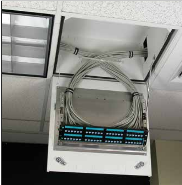
CZE Series Ceiling Enclosure with Ortronics® Patch Panel.
