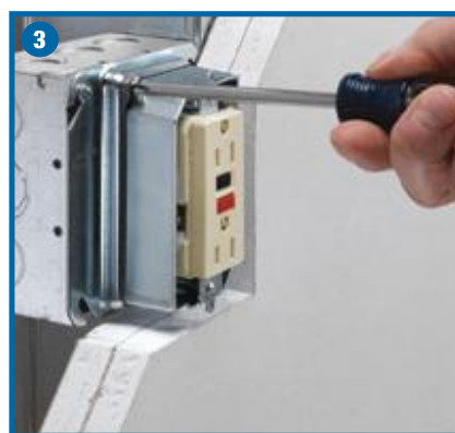
Re-tighten... Adjustment screws.
