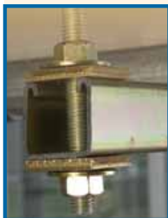
Standard method using nuts and washers
