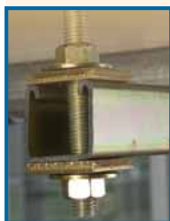
Standard method using nuts and washers
